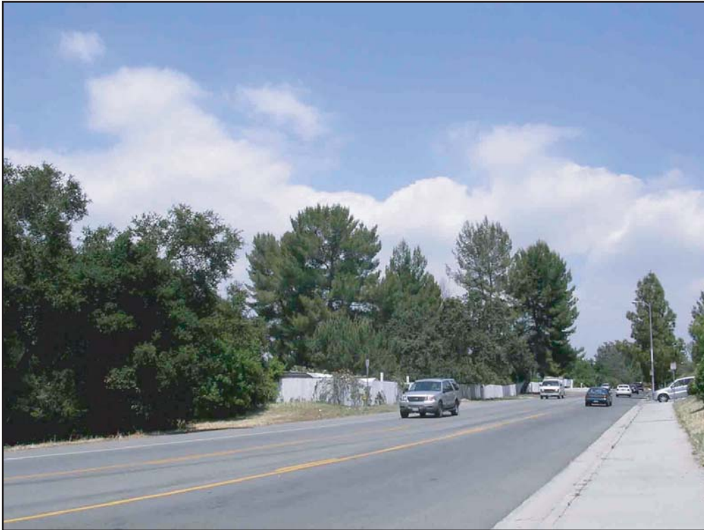
Photograph O: View looking east, across Mulholland Drive, at adjacent properties to the east of the Project Site.
