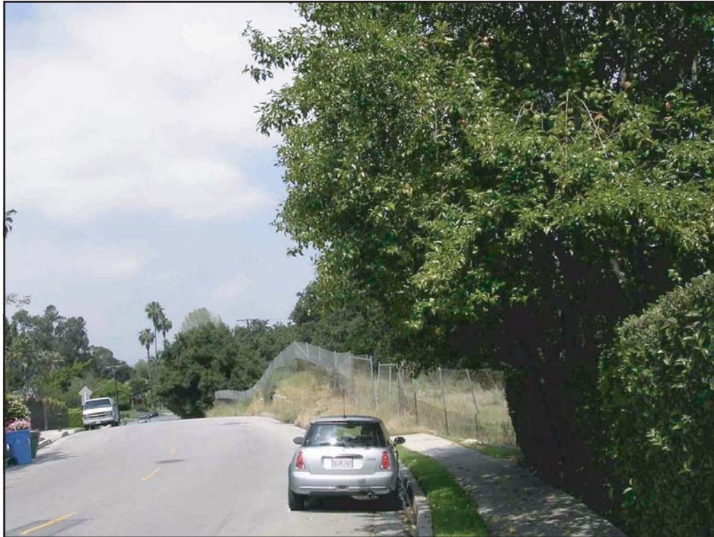
Photograph M: Poorly maintained site fencing and weedy growth along San Feliciano Drive.
