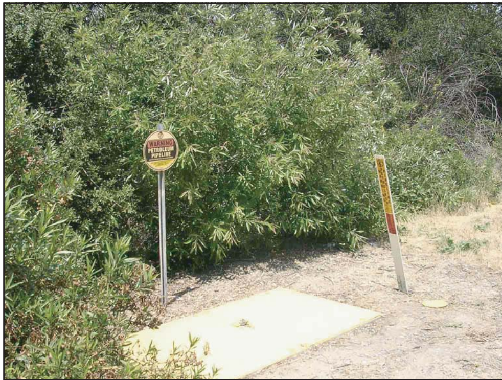
View 11: Gas line vault and warning signs on the north side of Mulholland Drive
